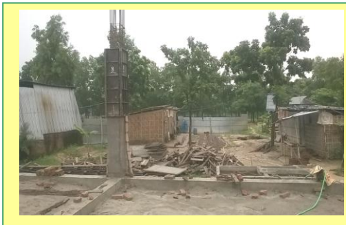
Picture-1 Construction camp and construction materials
